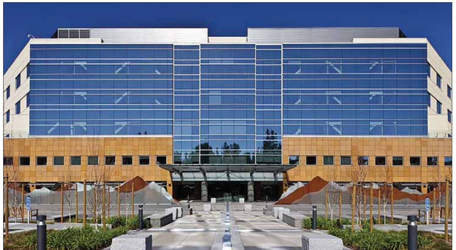
An exterior view of John Muir Health's Walnut Creek Medical Center. They have another hospital location in Concord and are in the process of acquiring San Ramon Regional Medical Center. COURTESY JMH
