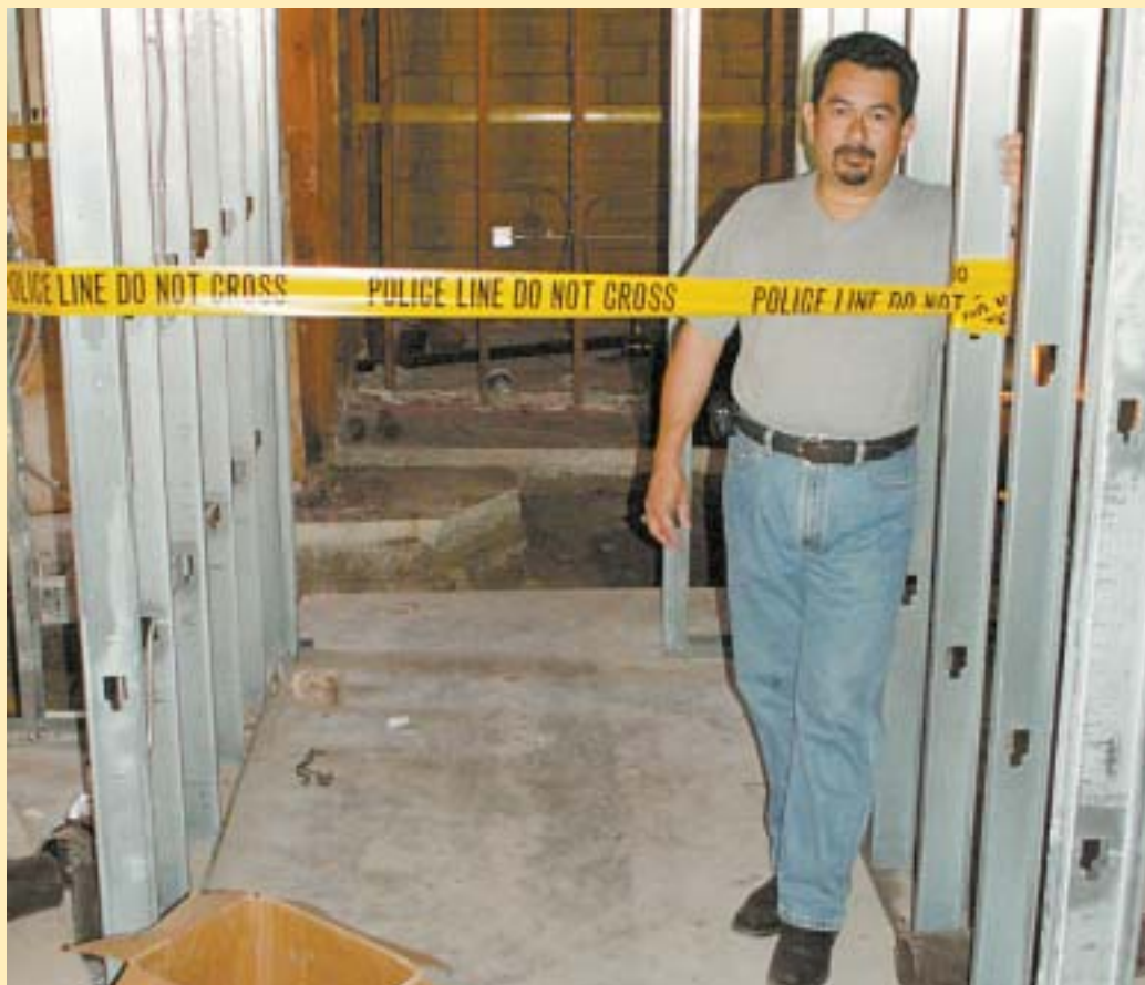
Andrew Galvan has been designated a "most likely descendent" of the local Bay Miwok Indians and is responsible for the bones found on Hartz Avenue as the former Country Waffles floor was being dug up to renovate for a new Mountain Mike's Pizza. Galvan said the bones will be reburied at the Ohlone Cemetery in Fremont upon project completion.
