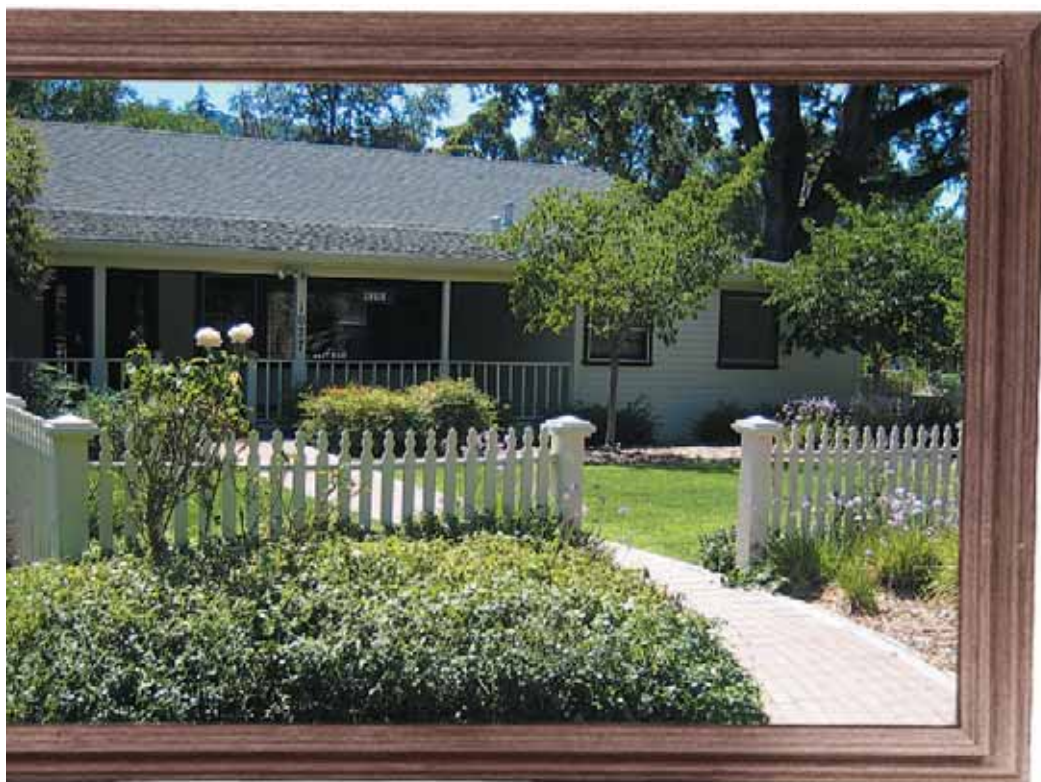
The Swain House, above, was built in the mid-1920s for caretakers, and is named after Ann and Capt. Isaac Swain, who gave money to the San Francisco Orphanage Asylum that enabled it to buy the land for a summer camp. The building now housing the YMCA offices was once the junior boys dorm.
