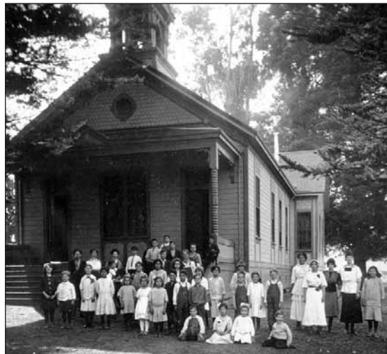
The second Alamo Grammar School, at the northwest corner of Stone Valley Road and Danville Boulevard, was remodeled several times. In 1904, 61 students were enrolled.
