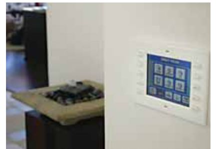
A six-inch touch screen controls the heat and music throughout the entire house.
