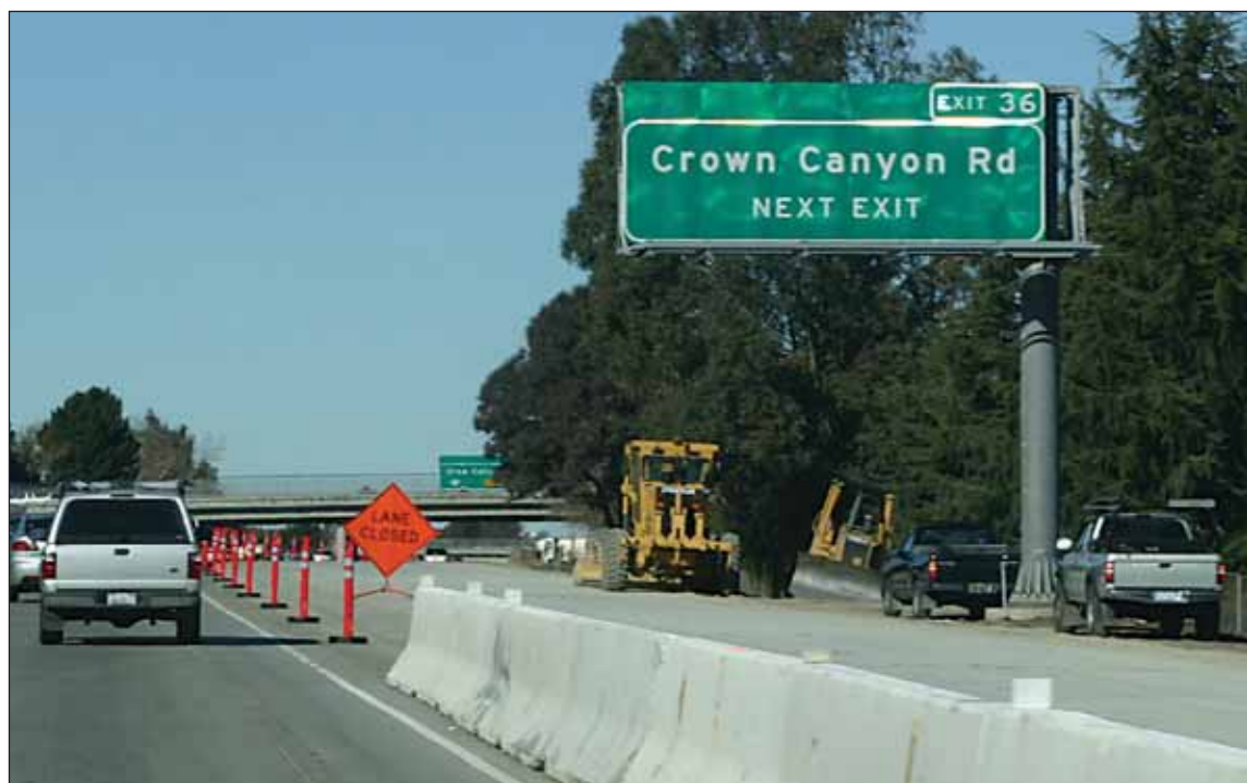
On Wednesday last week the freeway turnout to Crow Canyon Road took on a regal aspect. Caltrans corrected the sign later that day to read Crow Canyon Road.
