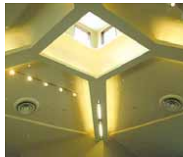
The ceiling of the new Beth Chaim Congregation synagogue.
