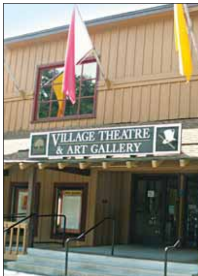
The Village Theatre on Front Street in Danville is undergoing renovations.
