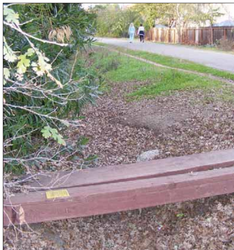
A footbridge near La Serena Avenue in Alamo allows its owners to maneuver over a dip in the landscape from their home to the Iron Horse Trail. It was yellow-tagged by the county as an illegal encroachment.
