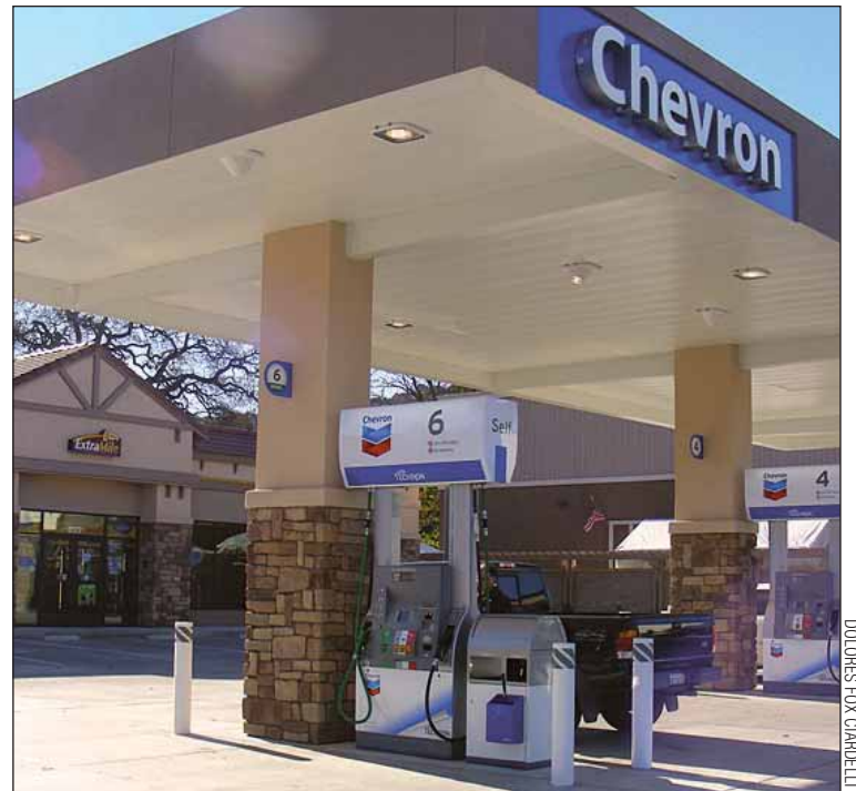
The renovated Chevron station is open for business in Alamo, with new fuel pumps and a large Extra Mile convenience store.
