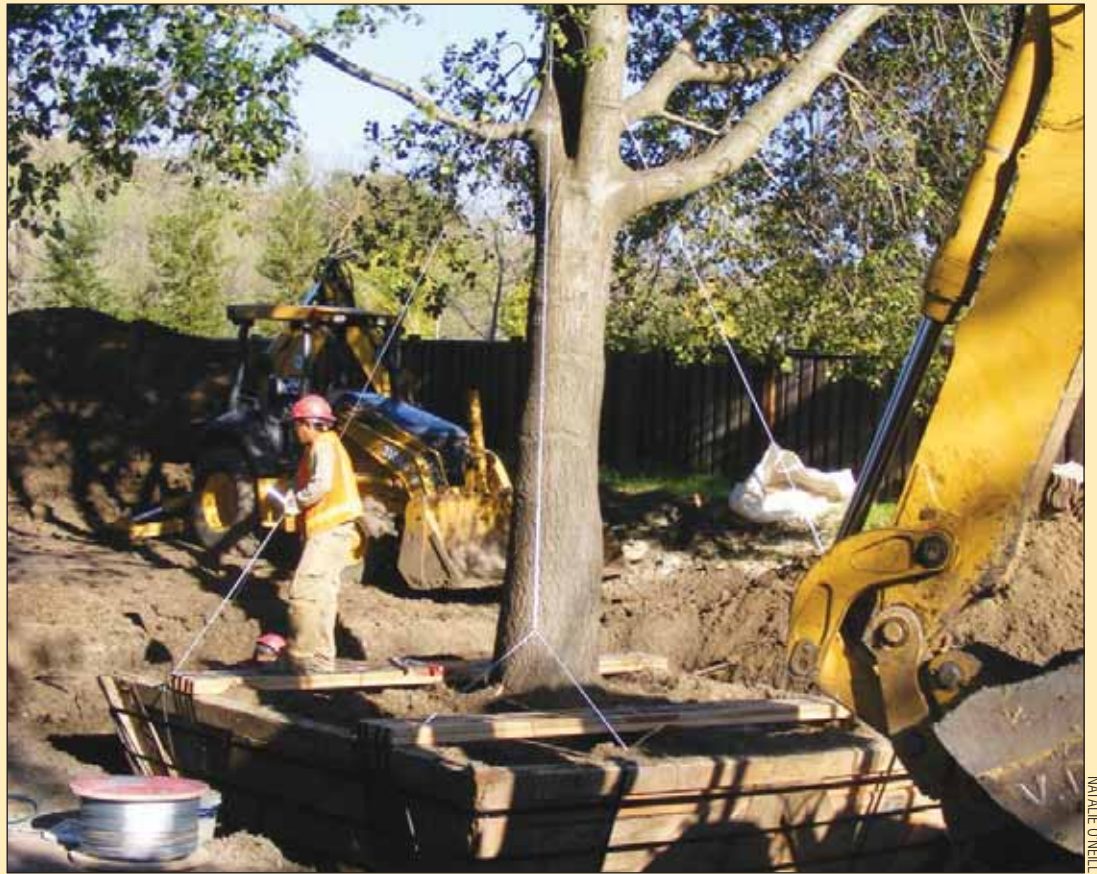
Workers are carefully boxing an oak tree to be moved by crane from the YMCA property in Alamo into a neighboring yard.
