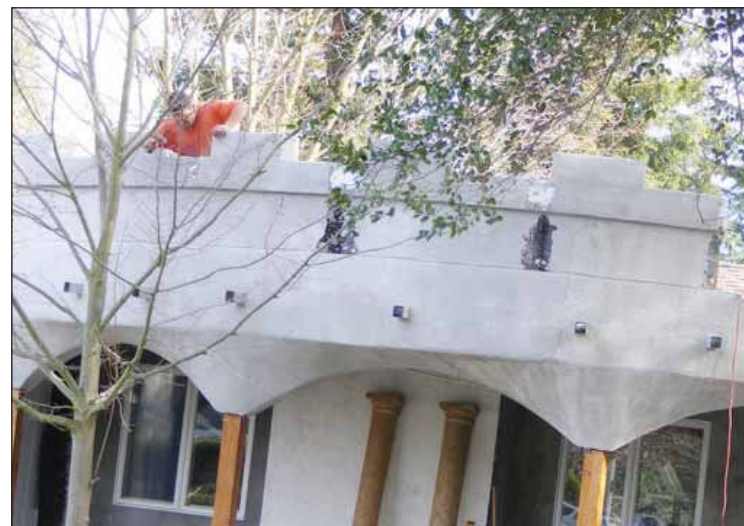
Workers in late February begin dismantling the Alamo castle on Hemme Avenue. Homeowner T.J. Baker, who designed the castle, has left town.
