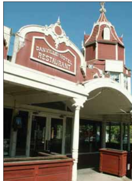
The old Danville Hotel Restaurant is the centerpiece of the Old West buildings that were built 50 years ago and are now being torn down for redevelopment. Plans call for three stories with eight residential condos on the second and third floors, commercial offices on the first floor facing the center quad, and underground parking.
