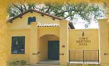
1989 - Mission-style church building on Front Street is restored by Danville and opened as the Town Meeting Hall.
