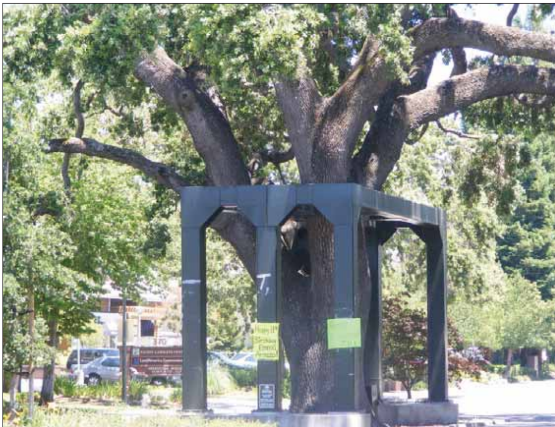
A steel structure was built around the Danville Oak in 2001 to support the tree, which is showing signs of decay in its old age.
