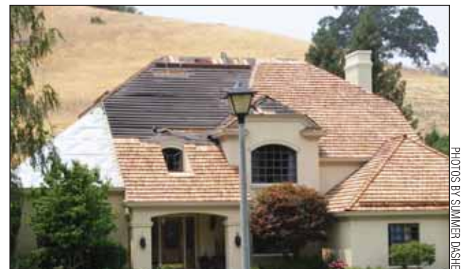
This wood shake roof in Bryan Ranch is being replaced with new shake, the only material currently allowed, except for tile.
