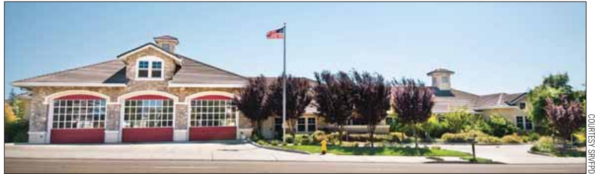
The new fire station of the San Ramon Valley Fire Protection District at 11445 Windemere Parkway in San Ramon.
